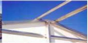
Tested framing system: 30-40 lbs. Snow Load 75-100 mph Wind Load
