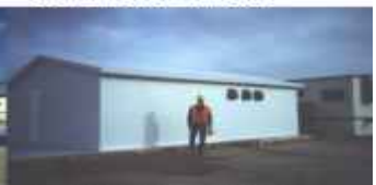
Building was delivered and erected in less than 4 weeks ARO.
