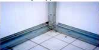
Galvanized Hat section on bottom provide additional panel support.
