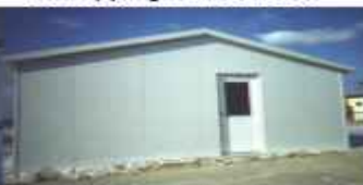
Capping around corners, ridge and around door openings are made of 26ga. Steel.
